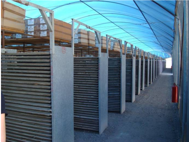
Copiapó core storage facility
